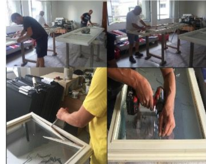
replacement of the existing glass with a new one
