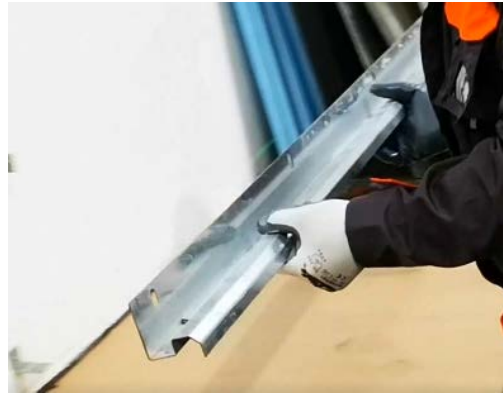
Horizontal profile starting of the system
