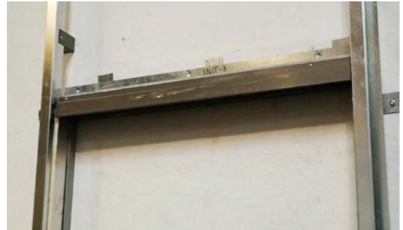
Lintel metallic sheet finishing
