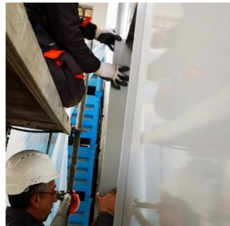
Jamb metallic sheet finishing
