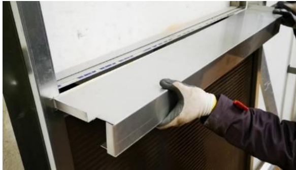
Windowsill metallic sheet finishing
