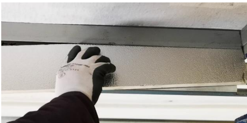
PIR boards (balconies, jambs, lintels, windowsill)
